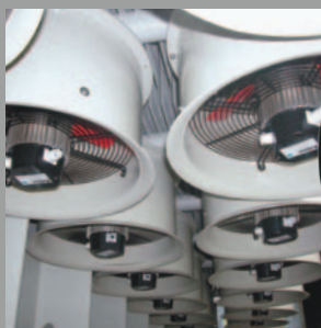
High voltage transformer.
